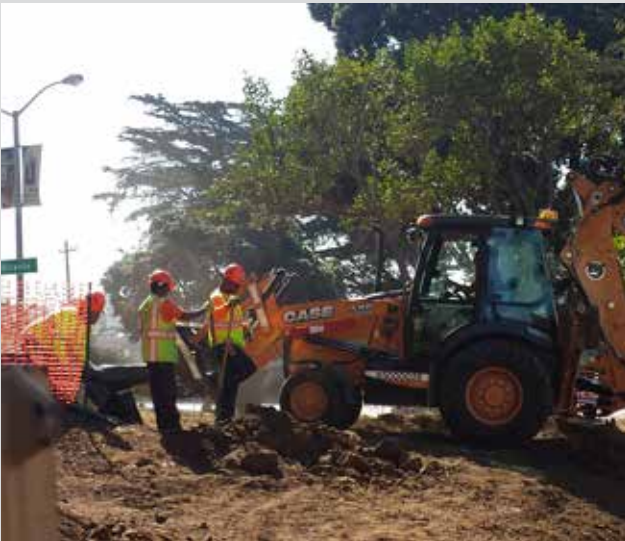
Sunset Blvd Greenway/Sunset GI Early Implementation project breaks ground.
