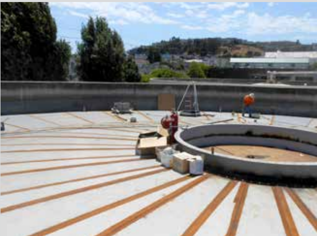
Welding rooftop panels on Digester #7, Southeast Plant (SEP)
