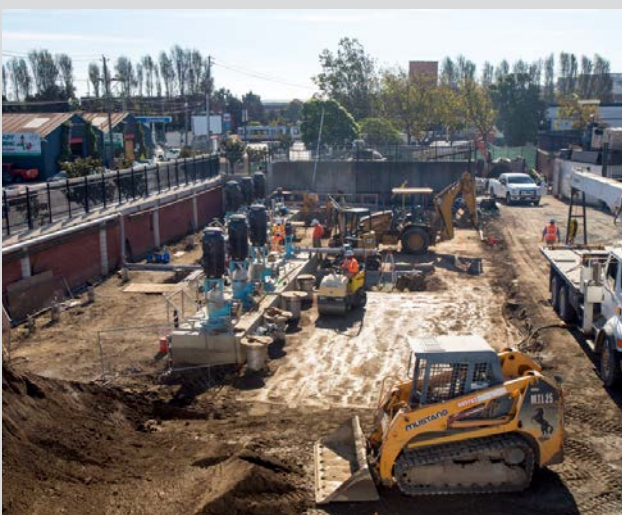
SEP 521/522 and Disinfection Upgrades, site of sump pump motor pipe supports.
