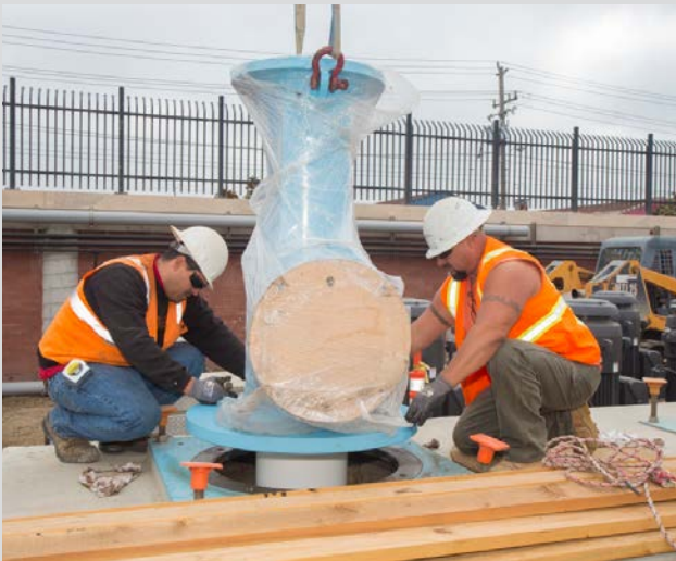
SEP New Piping System, Vertical Turbine Pump installation
