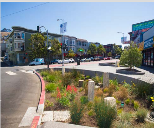
Completed construction of Mission & Valencia Streets Green Gateway
