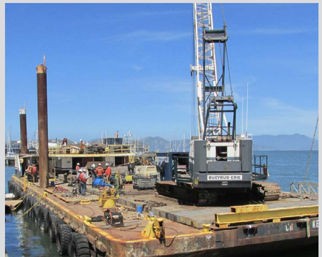
North Point Outfall Rehabilitation sediment removal
