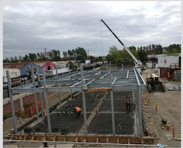
Building 522 construction at SEP
