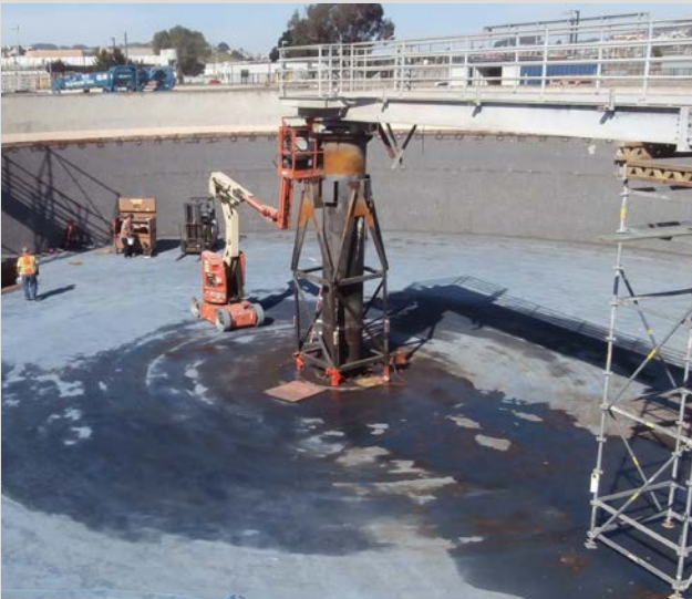
SEP Secondary Clarifier No. 6 catwalk and tower removal.
