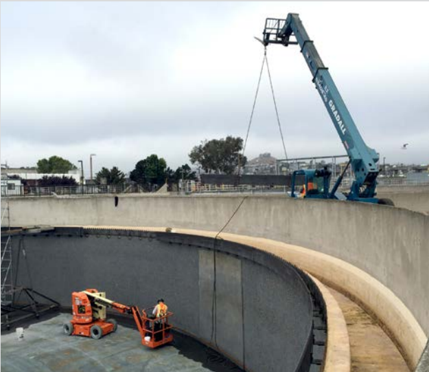
SEP Secondary Clarifier No. 6 effluent weir removal.
