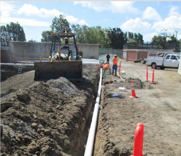
Site dewatering piping installation for the SEP Building 920 location.
