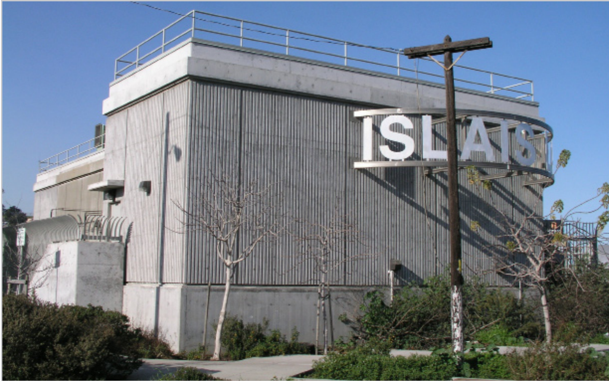
Figure I-17. Booster Effluent Pump Station
