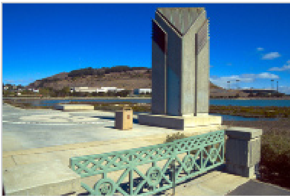
Figure I-15. Sunnydale Pump Station
