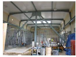
Interior seismic and tenant improvement work at the Lake Merced existing pump station building
