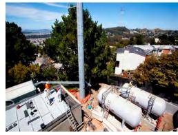
Construction of Forest Hill Pump Station and Hydro-pneumatic Tanks
